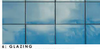
6: GLAZING GUARDIAN GLASS & STOREFRONT SYSTEM CLEAR, LEANING SLIGHTLY BLUE/GRAY
